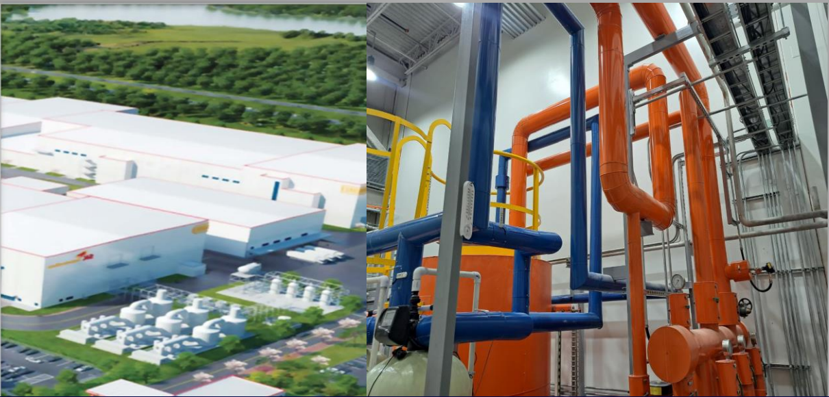
HOT OIL PIPE, HVAC INSTALLATION in Electrode Area
