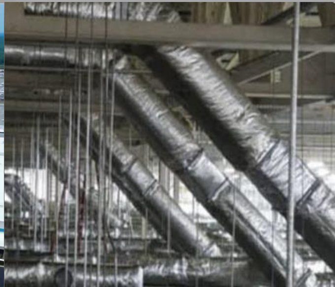
CLEAN ROOM DUCT SYSTEM INSTALLATION
