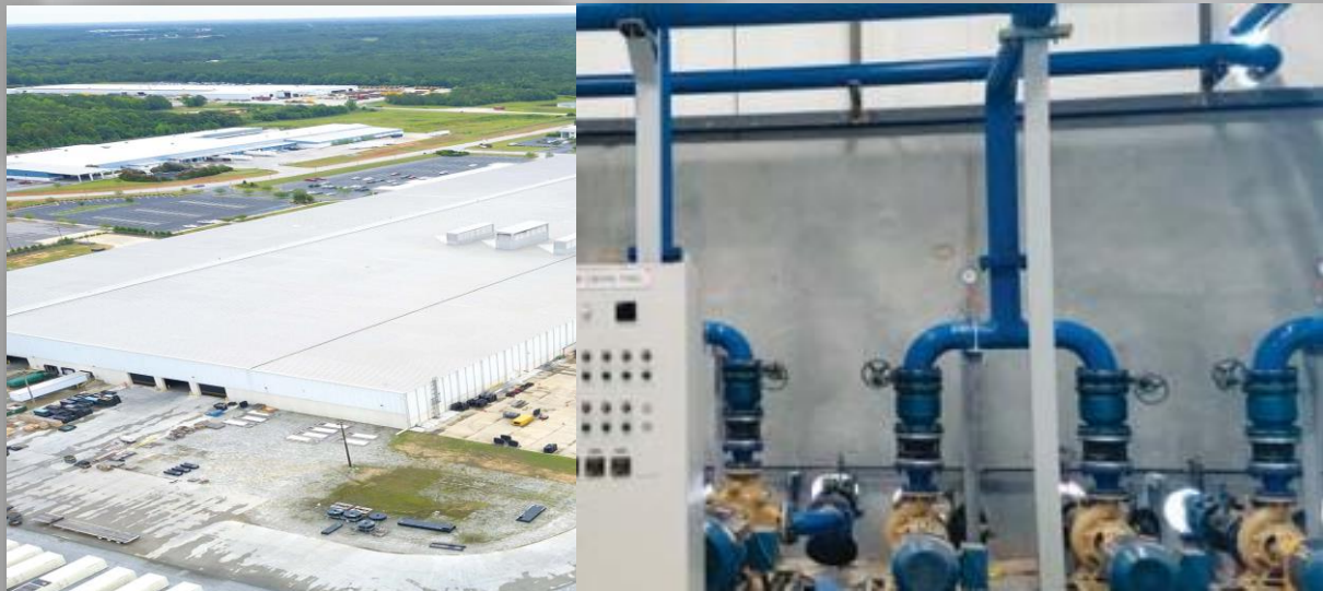
COOLING WATER PIPE INSTALLATION
